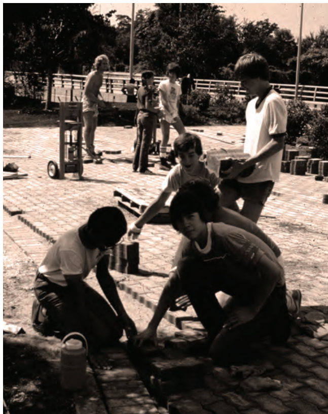
Volunteers Lay Bricks - 1981
