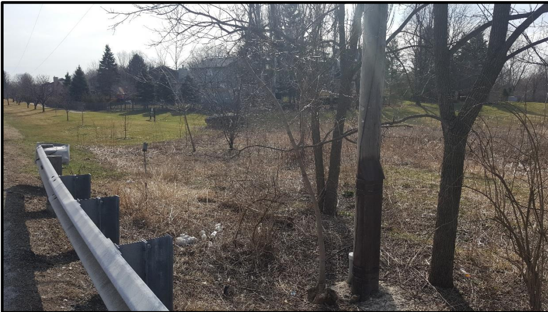
Photograph 2: SE bridge corner looking at southern ROW and Naperville Park District land
