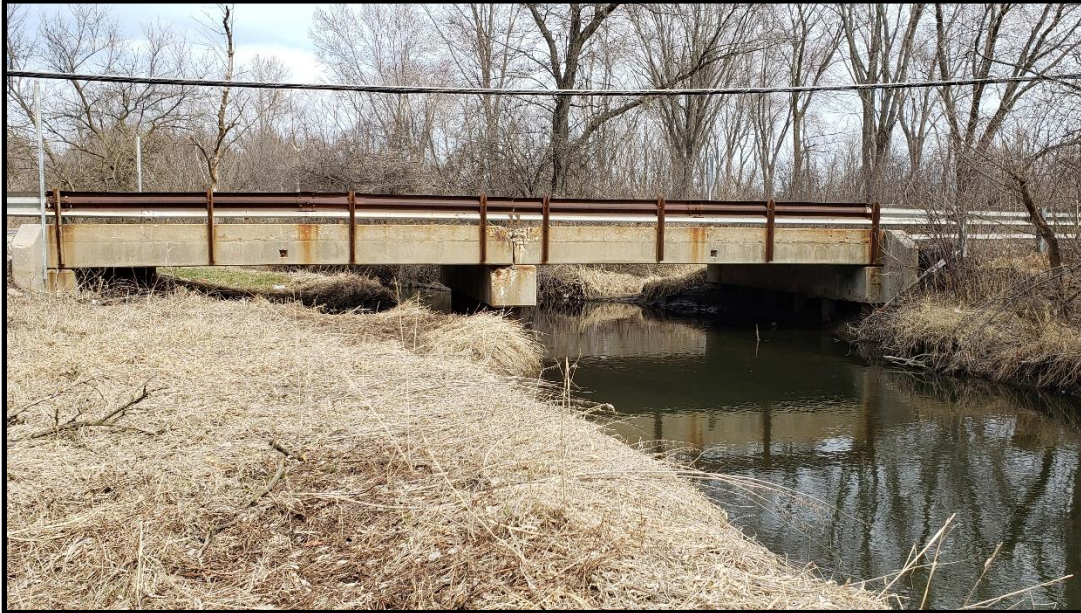
Photograph 1: Looking north at the south face of the bridge
