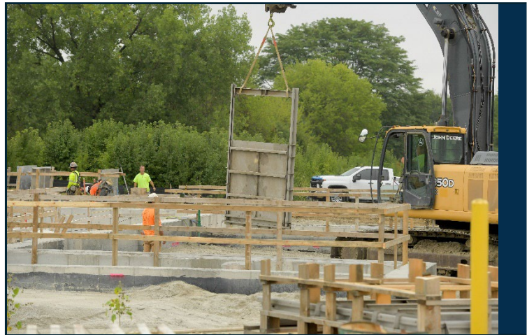
Springbrook Water Reclamation Center capital improvements are underway to address regulatory requirements as well as aging infrastructure and capacity.
